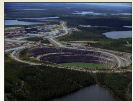
AREVA's JEB Mill and Tailings Management Facility.
